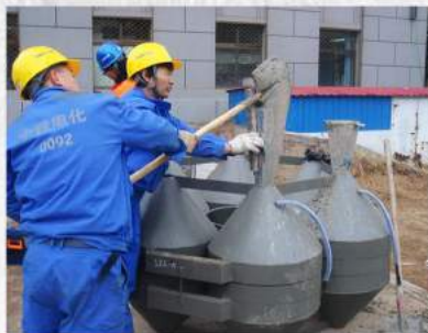
Precast of flow guides
