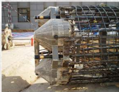
Weld Super Cell to the cage
