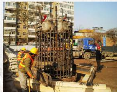
Install the rebar cage
