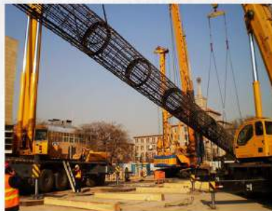
Lift the cage with Super Cell
